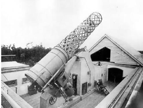
**The Great Melbourne Telescope (GMT) installed in the GMT house at Melbourne Observatory 1885.**
